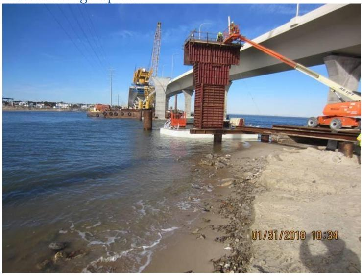
The concrete pour over the weekend that caused the Lesner Bridge to be reduced to one lane each way broke a logjam in trying to get the eastbound span's superstructure across Lynnhaven Inlet. About 400 cubic yards of concrete were poured for Pier #5 The photo here shows forms being removed from Pier #7looking westward across the inlet.
