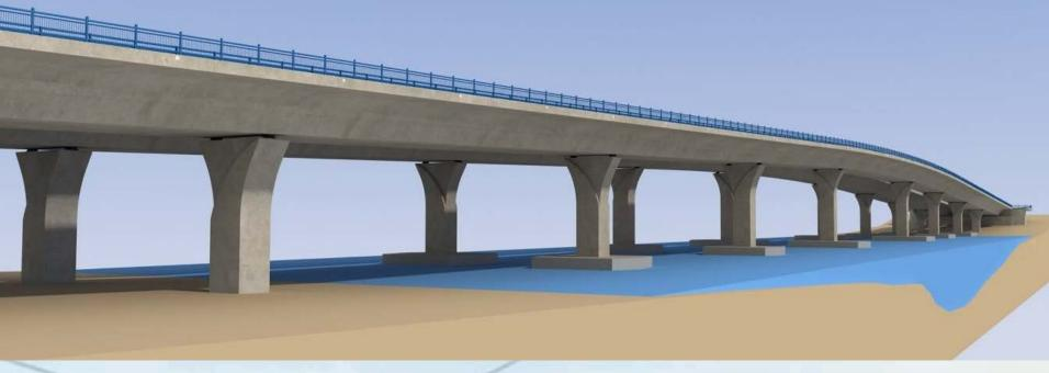
All visible surfaces of box girder, piers, footings, abutments, barriers, curbs & MSE walls to be stained per specifications – stain color same as local beach sand.
